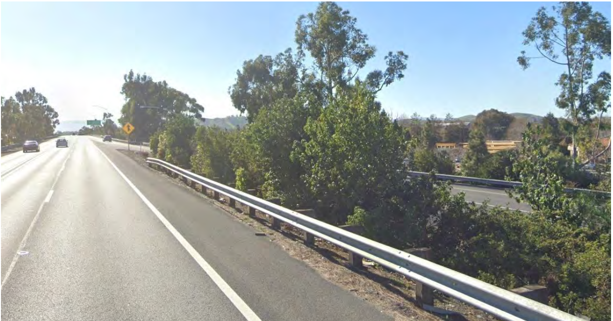
Figure 3.2-8. Viewpoint A – Ardenwood Park and Ride from SR 84, looking southwest (Proposed Project)
